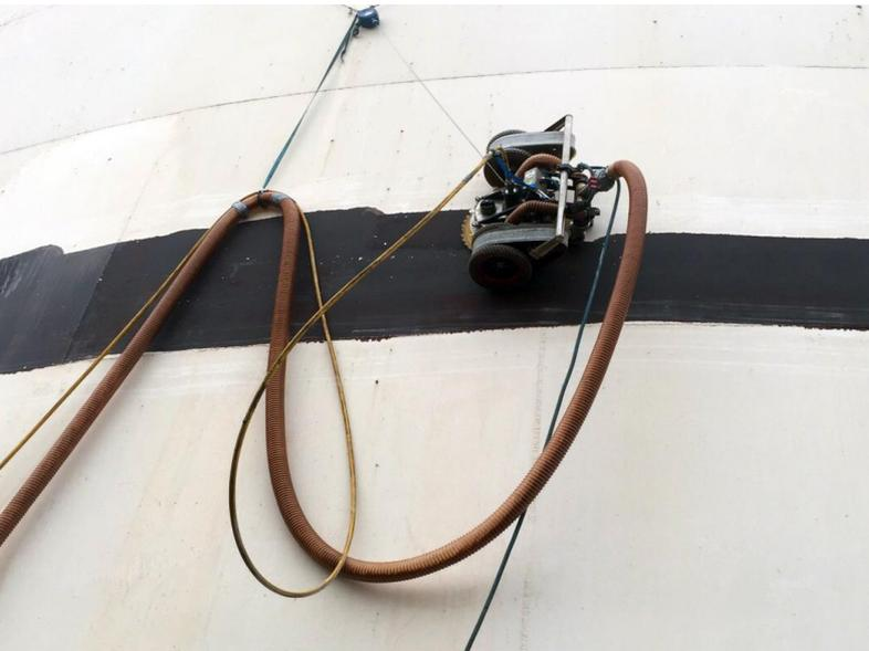
▲ The outside of a tank is hydrojetted, with the waste water collected by a vacuum unit
